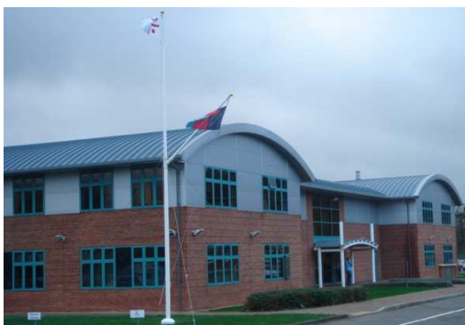
The UK's flagship Joint organisation Headquarters at Shrivenham, Wiltshire
